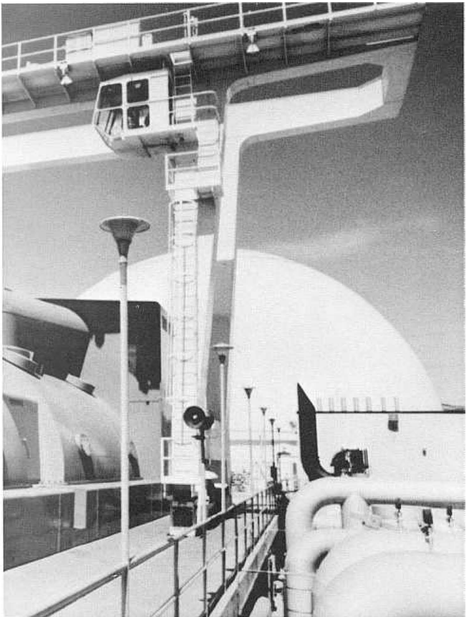
The nuclear generating station at San Onofre, California, is a forerunner of hundreds of similar facilities now under construction to help the U.S. meet the growing energy crunch.
